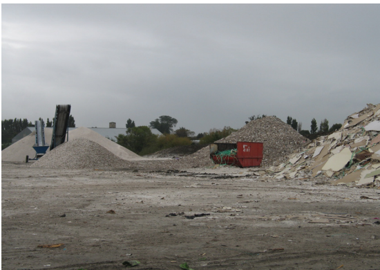
Processing Plant at Crusaders Landscaping, Christchurch.
