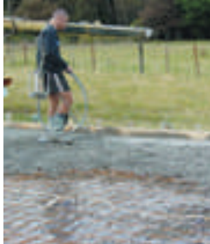
The slab edge thickening is being vibrated: take care, on the main area of the slab, to ensure the vibrator does not slip through the mesh and damage the DPM.
