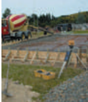
The concrete is being spread: a laser level gives accurate levelling.
