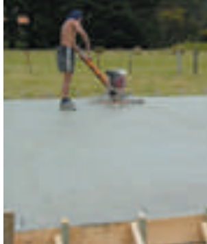
After the initial 'set', a rotary power float is used to give a high-quality finish.
