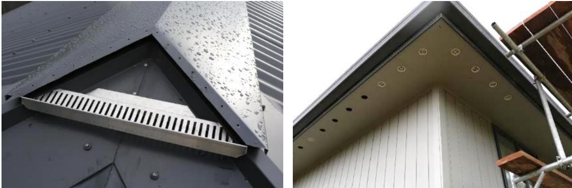
Figure 2. Ridge cap and soffit vents installed at the National Park building.
