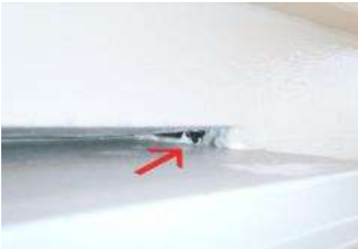
No sealing at the end of the head flashings
