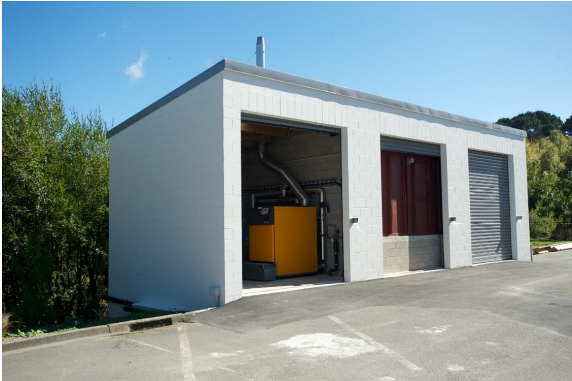
Figure 6 The new wood pellet boiler (left) and the hopper (centre)
