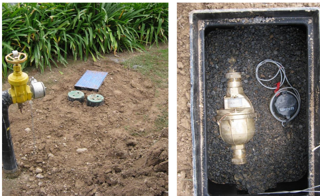
Figure 14 Water metering for the Fire and Structure Lab's and the Kauri building
