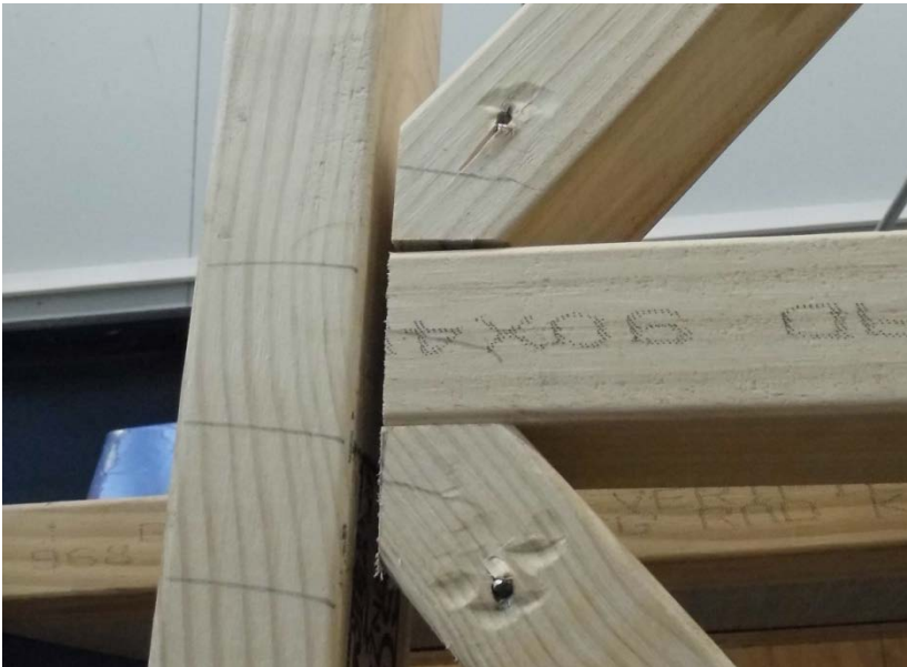
Figure 39. Gaps opened at intermediate joints in Brace 4 during testing after strengthening
