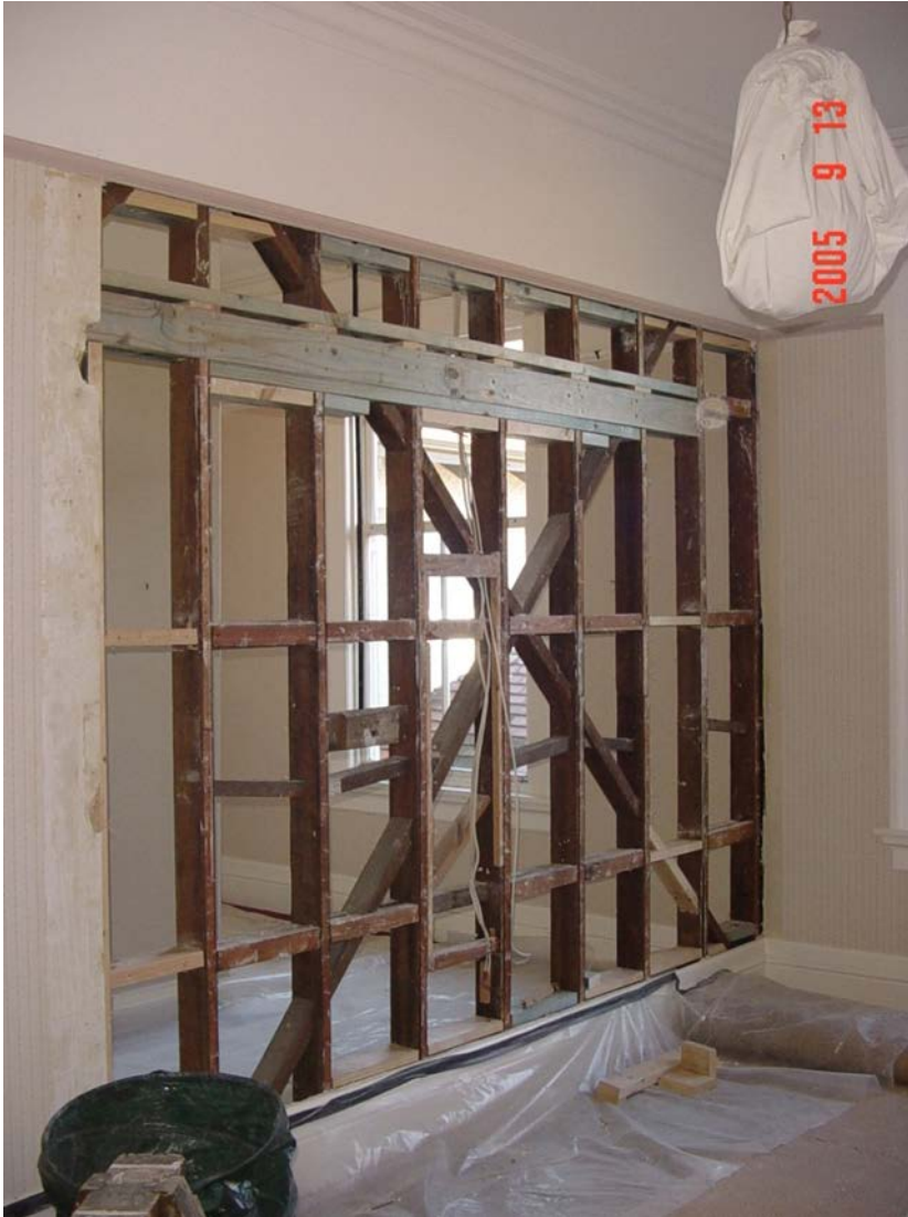
Figure 7. Wall 1 framing in the insitu fibrous plaster wall tests
