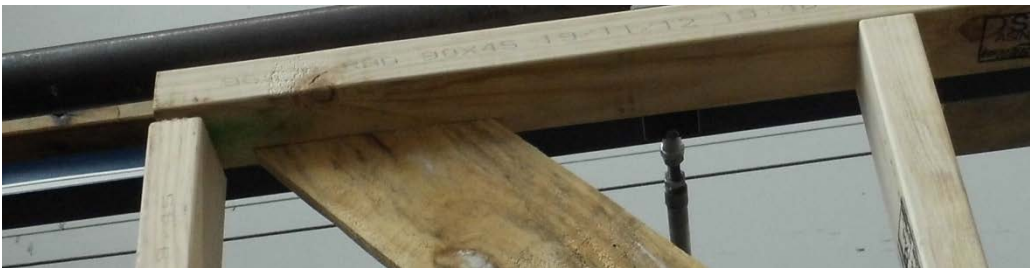
Figure 16. Diagonal brace lifts top plate in tests before connection strengthening
