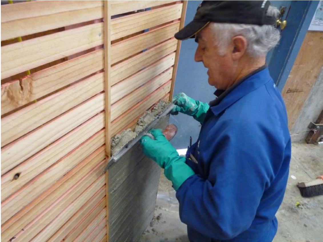
Figure 10. Applying plaster to the lath and plaster test wall
