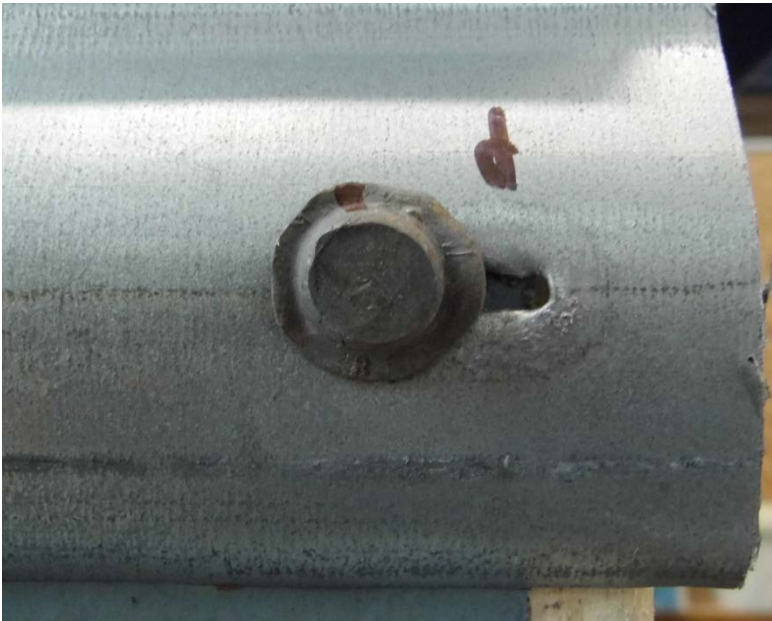
Figure 61. Lead-head nails used for Sheet 4 and Sheet 5
