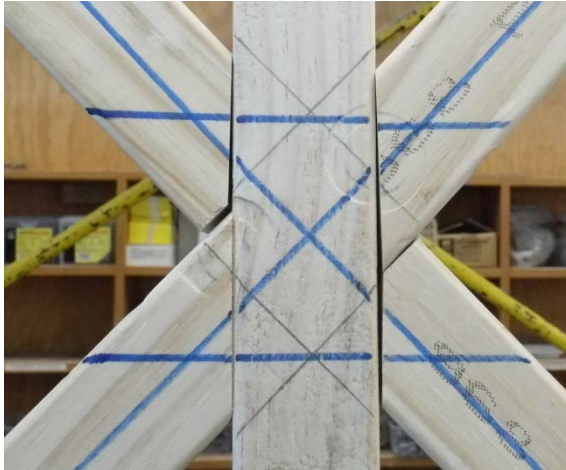
Figure 35. Little joint movement occurred at the intersection of diagonal braces (photograph taken at same stage as Figure 34)
