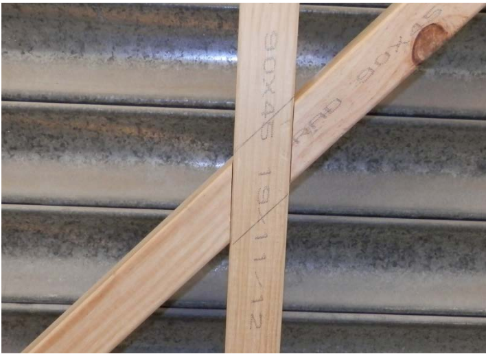
Figure 22. Centre joint in specimen for single diagonal braces cut between studs
