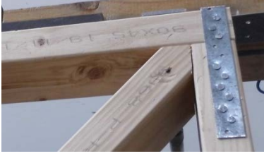
Figure 38. Strengthening used in Brace 4
