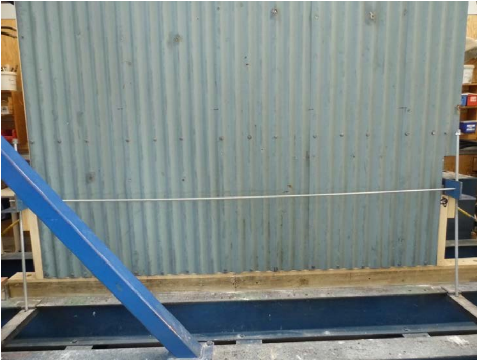
Figure 66. Views of pattern of lead-head nails – horizontal corrugated steel
