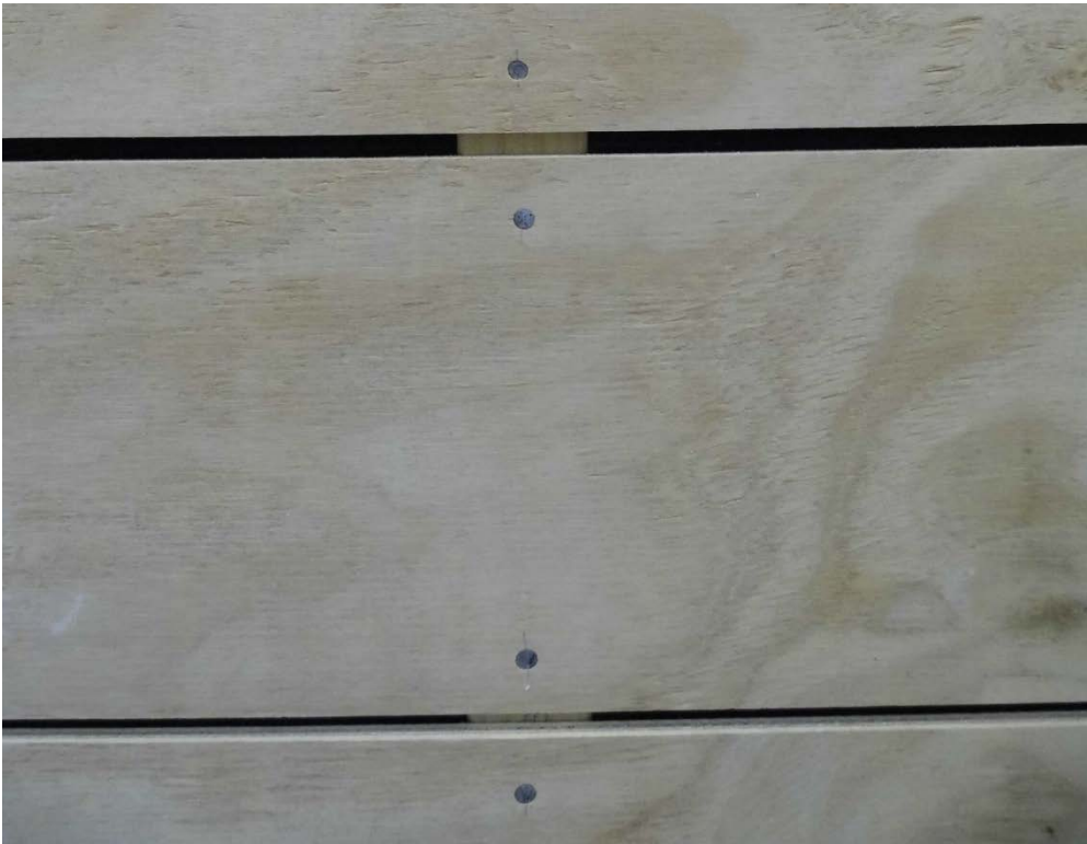
Figure 43. Nailing at stud for horizontal boarded wall
