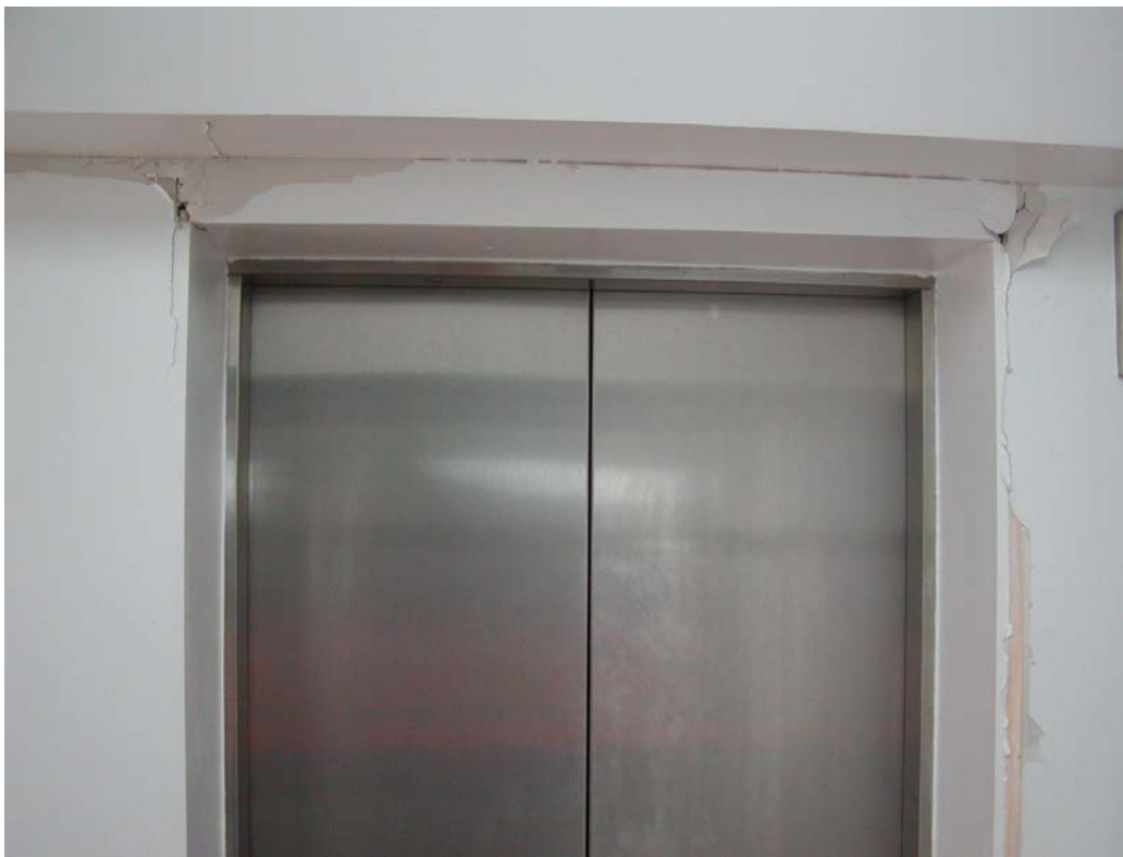
Figure 19: Cracking of plasterboard surrounding an elevator doorset
