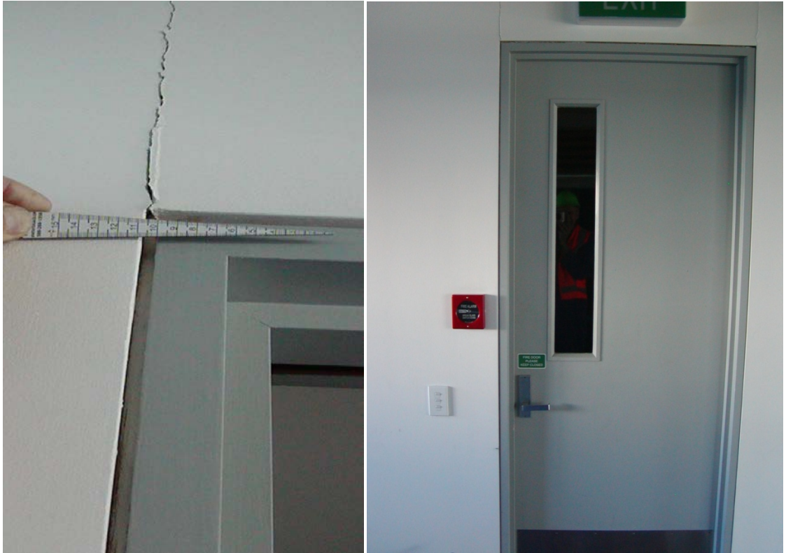
Figure 13: Vertical crack on plasterboard above door frame and 7 mm gap between plasterboard and door frame
