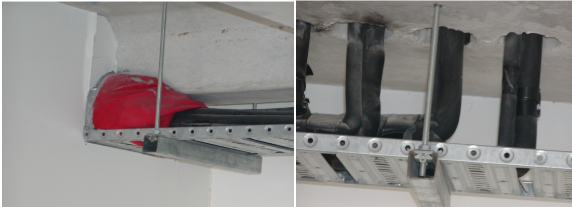
Figure 9: Service penetration through lobby firewall and floor above
