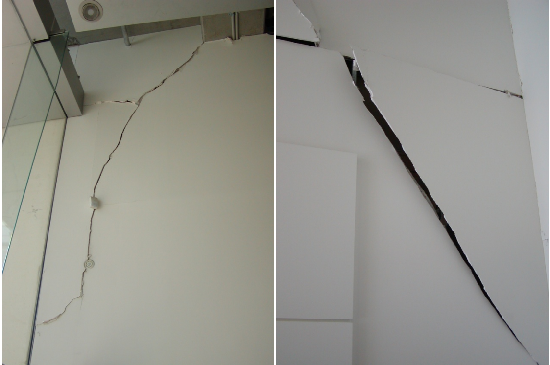
Figure 6: Severe cracking at opposite ends of the 30/30/30 firewall inside the entrance lobby
