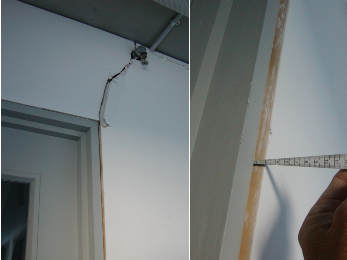
Figure 12: Cracked and displaced lining on stairwell side of door frames
