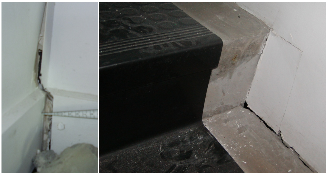
Figure 15: Stairwell plasterboard damage in corner and on stair tread
