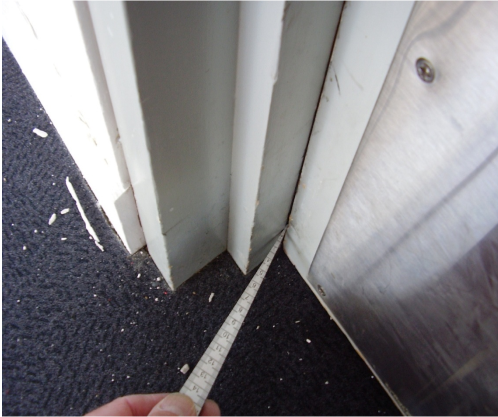
Figure 11: 1.5 mm gap between door stop and leaf
