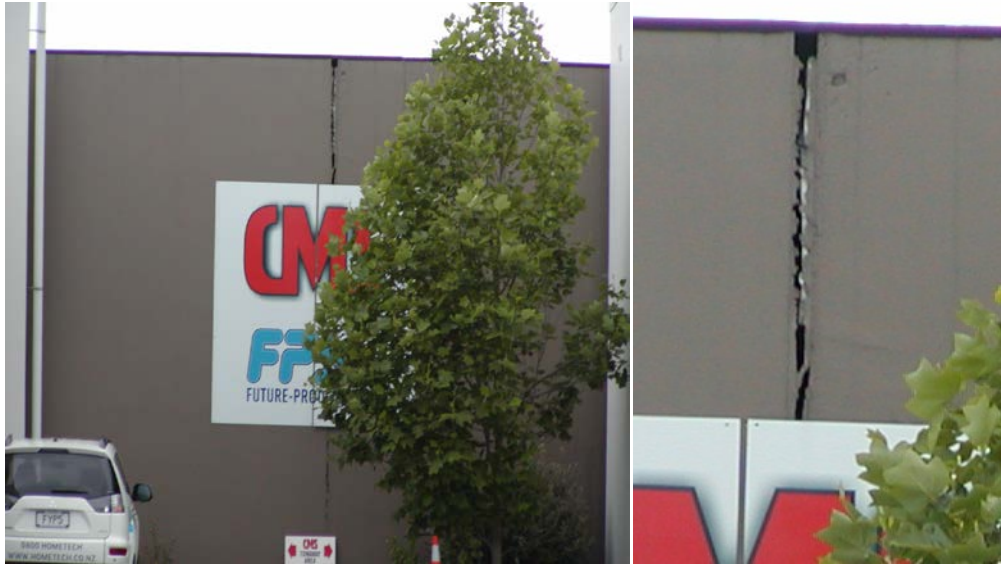
Figure 22: Typical opening of butt joints in concrete tilt slab panels
