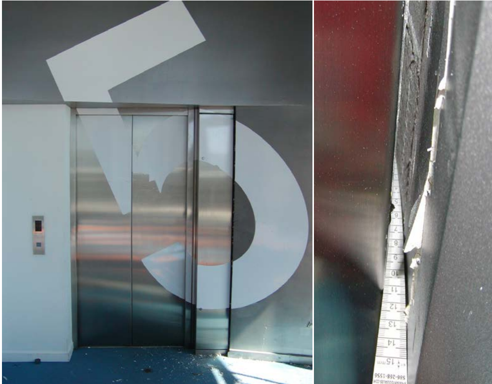
Figure 18: Top floor elevator doorset and 10 mm gap on right hand side
