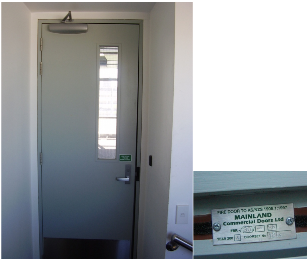
Figure 10: Fire door between stairwell and floor, -/30/- SM view from the stairwell side, intumescent strip is included to achieve smoke control
