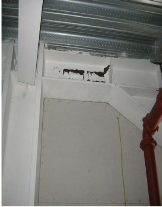
Figure 23: Loss of intumescent paint on steel beam post-earthquake
