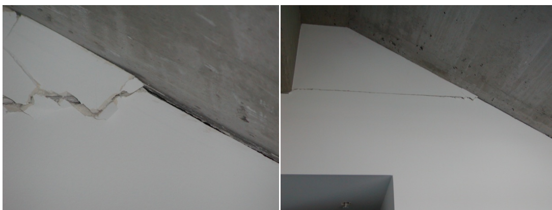
Figure 16: Plasterboard damage under scissor stair flight
