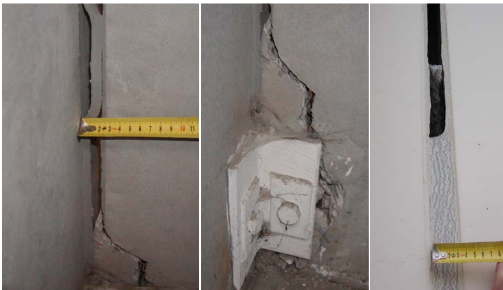
Figure 21: Internal corner and external butt joint
