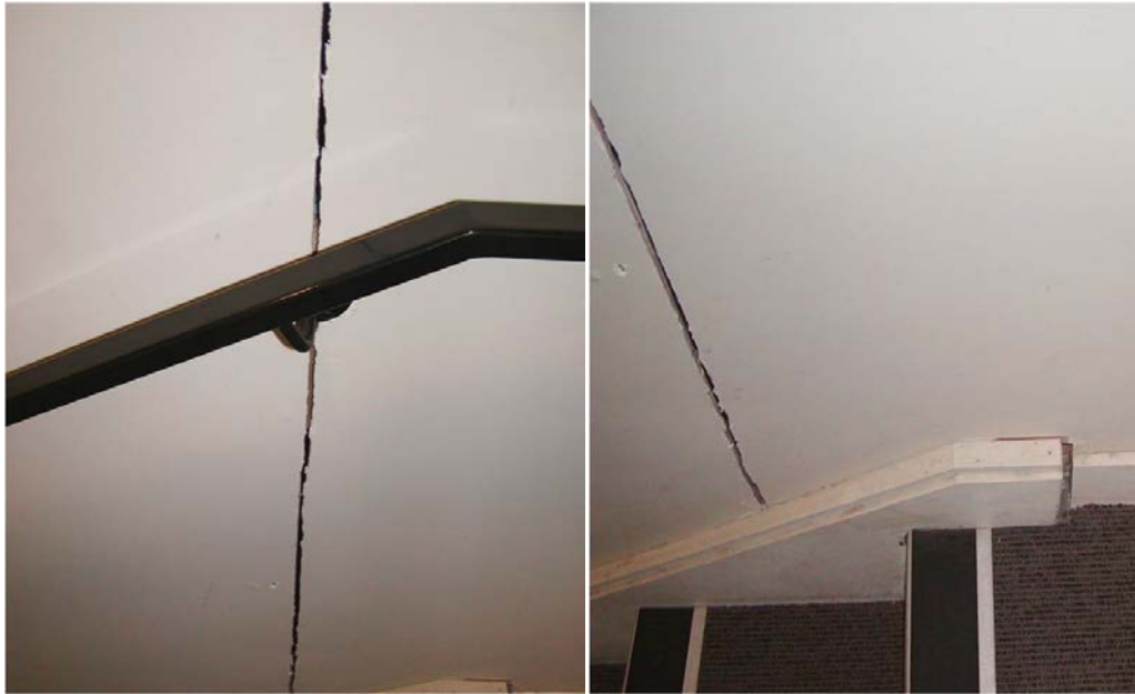
Figure 17: Vertical crack of ~4 mm at lining junction over double studs and opening of gap between stair flight and wall
