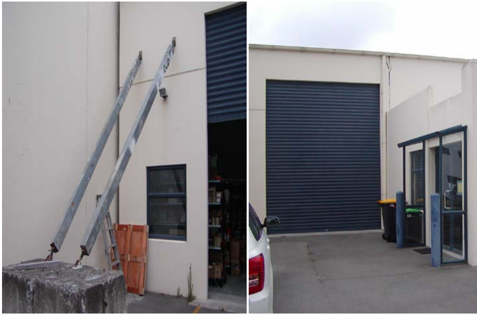
Figure 20: External view of typical concrete tilt slab building
