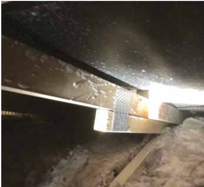
Mould growing on roof framing timber and roofing underlay in an Auckland house.
