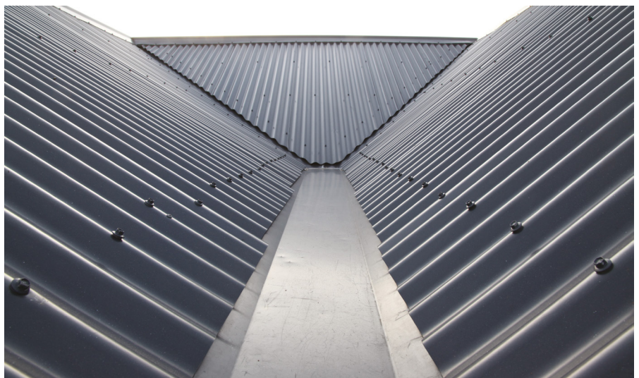
Internal gutters can deteriorate faster than the rest of the roofing and are difficult to repair.
