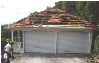
Tiles that are not appropriately fixed can be easily dislodged in an earthquake or by wind.
