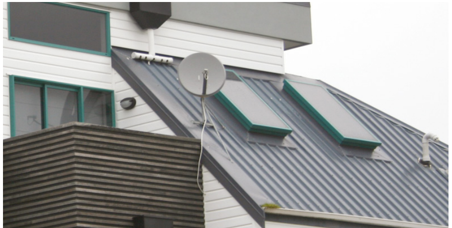
A relatively simple roof made complex by a wall cladding junction, a downpipe discharging from the roof above, penetrations, a satellite dish and multiple rooflights.
