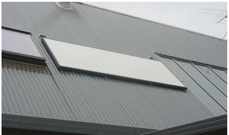
Roof-mounted items like solar panels must have a gap under them. If fitted tight to the roof, this may accelerate deterioration of the roofing under them as the surface cannot be accessed for maintenance.
