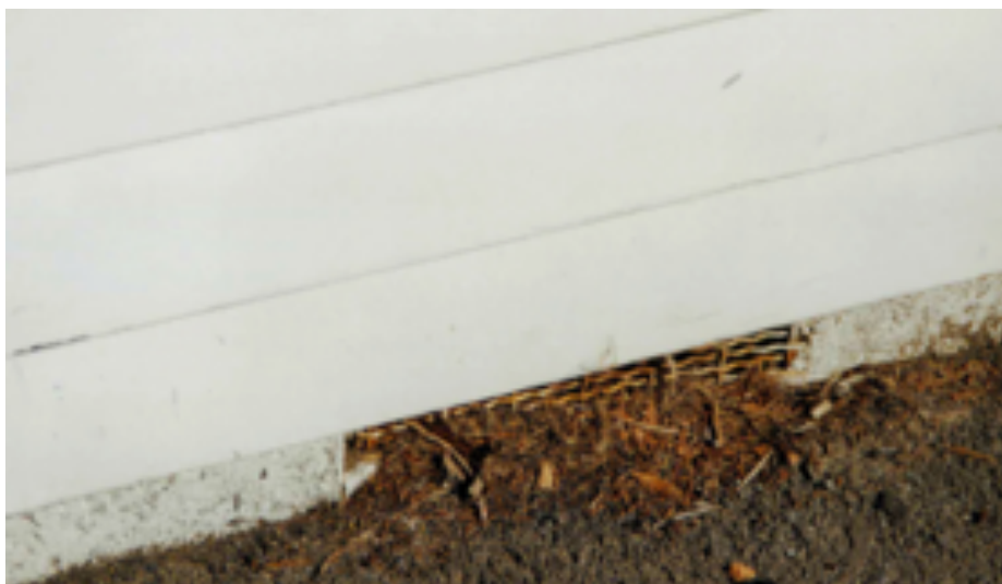
Subfloor vents are one of the house components most likely to be assessed as being in poor or serious condition.
