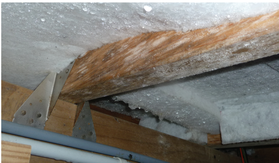
Poor subfloor ventilation can lead to problems with excess moisture.
