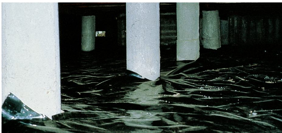
Installing a polythene ground cover under a house can reduce subfloor moisture levels.
