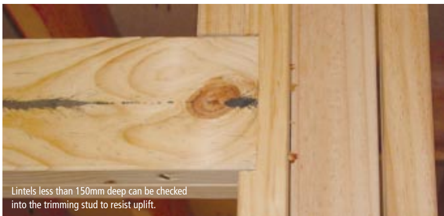
The top plate is fixed to the lintel and the lintel is fixed to the doubling stud.
