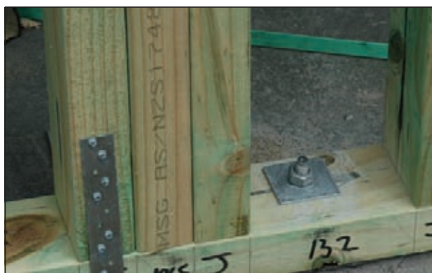
Figure 1 H3.1 may be dyed green or left uncoloured and continuously branded along the sides while H3.2 is not dyed. Both are required to have end marking. This structural use of H3.1 timber is acceptable as the framing will be protected from the weather.
