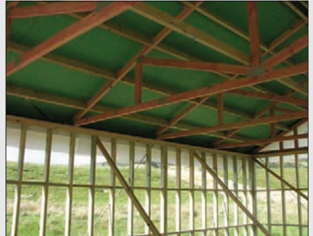
Figure 2 Underlay is an important part of the roof installation and should be installed tightly over netting.
