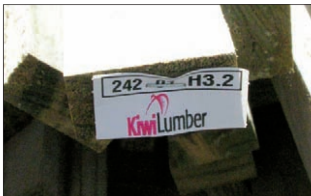
Figure 2 Batten clearly identified by end marking. Every length of timber is required to be identified.
