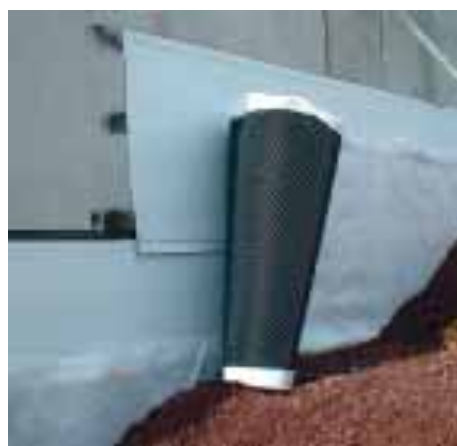
Figure 3: Drainage mat applied over tanking (photo courtesy of Maccaferri NZ Ltd)
