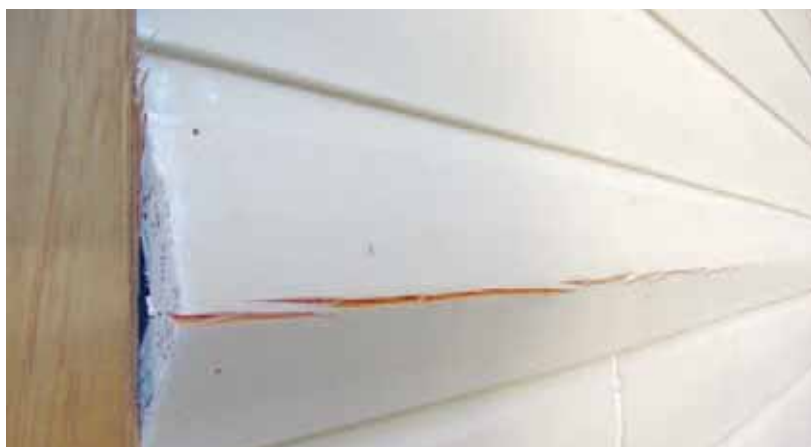
Figure 1: The cause of these badly cupped weatherboards can be seen in the lack of adequate expansion gaps at the top of each board.
