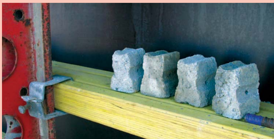
Concrete spacers are ideal for in-situ concrete walls.
