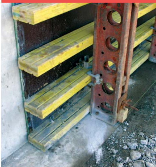
Through- and holding-down bolts in place.
