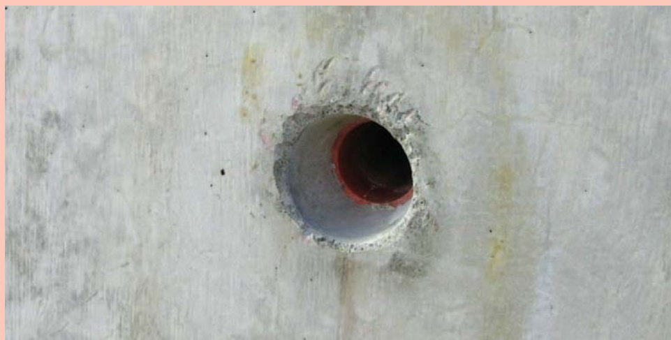
After stripping there may be holes to grout. Note the high quality concrete finish.
