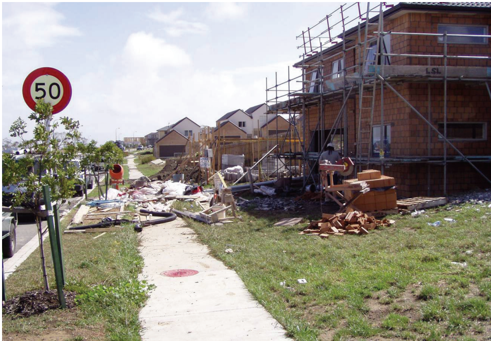
This Auckland building site looks like a tip – and it's putting both site workers and passers-by at risk. At least the site has appropriate roof edge protection.
