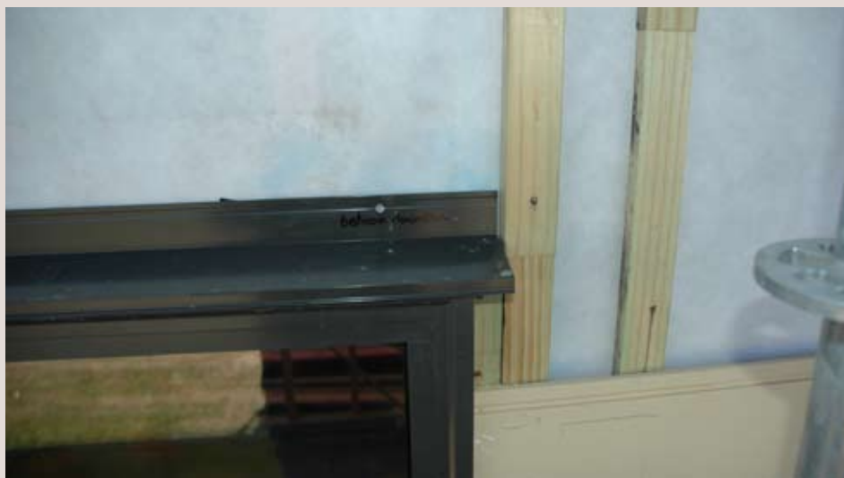
This construction has no stop-end and not enough cross-fall.
