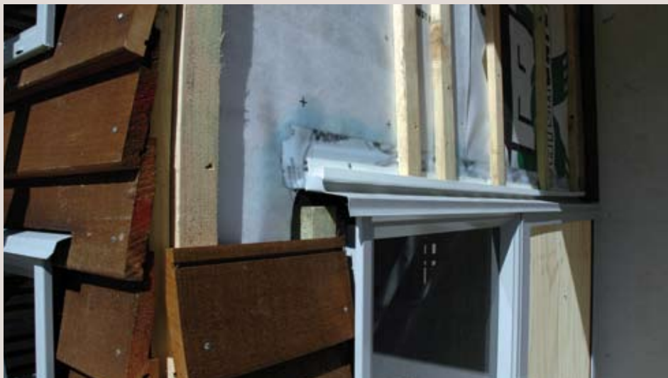
This building has stop-ends, but the cross-fall may not be enough.
