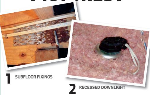
2. Insulation has been installed hard against this older style recessed downlight. This is a potential fire hazard as it could lead to overheating – the insulation should be 100 mm away from the fitting. I. There is very clear corrosion in these subfloor fixings, a nail plate and z nail. This indicates a potential problem with excessive subfloor moisture, or a lack of subfloor ventilation. The cause of the problem needs to be addressed.
