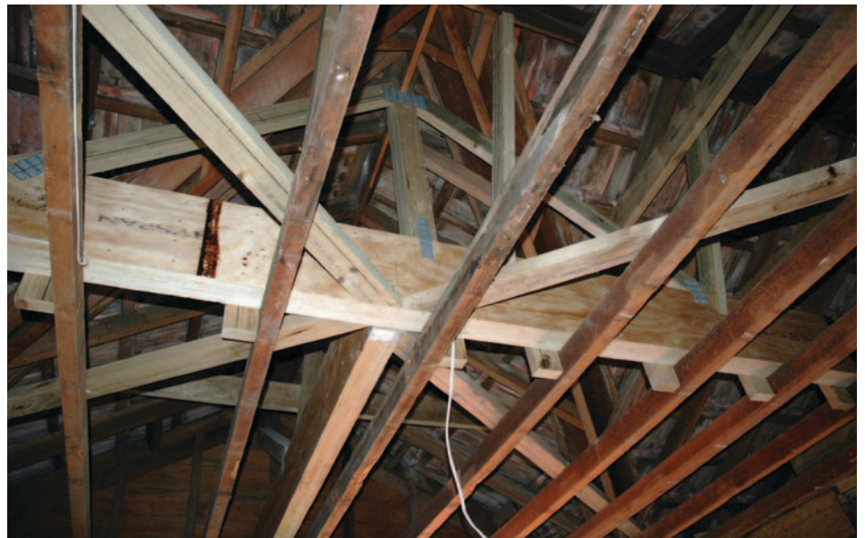
Figure 2: New structure supporting existing ceiling joists and ridge.
