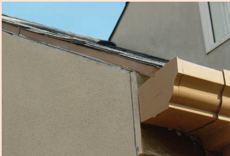
Figure 1: Unsatisfactory detail of stucco cladding butted up to timber blocking with no attempt at waterproofing the junction between the wall cladding and the asphalt shingle roofing.
