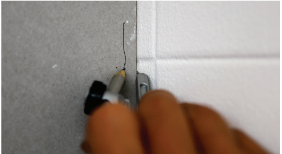
Scribing with a compass involves running the compass point along the irregular surface and marking the shape on the material to be cut.
