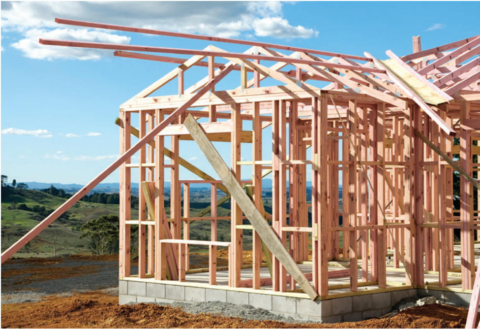
Making sure minimum ground level requirements are met and framing is straight and plumb will help the job run smoothly.
