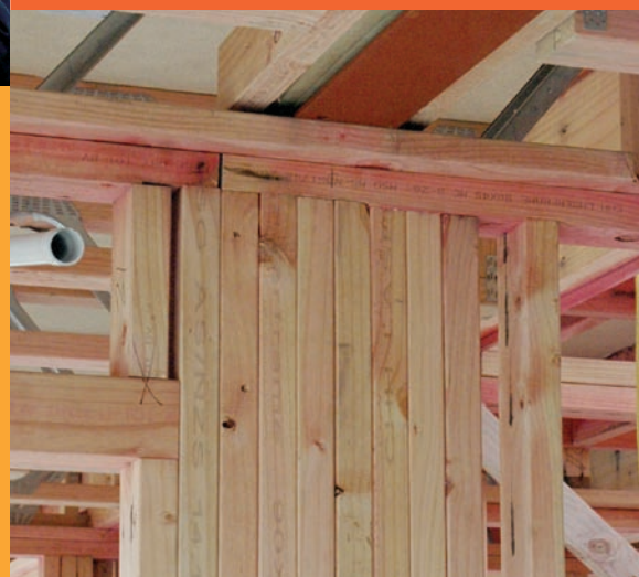
A typical top plate joint where the joint is not centred on a stud. Such joints require blocking, but in this case, the laminated studs supporting the steel beam above are providing support to the joint. However, the number of studs laminated together is outside the scope of Section 2.4.4.7 of NZS 3604.
