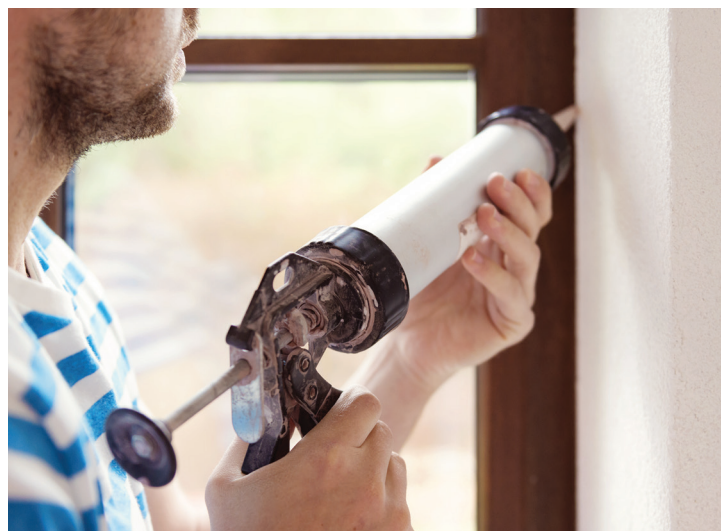
Figure 2. Push the sealant into the gap, moving the sealant gun forwards over the extruded sealant – do not pull the sealant gun.
