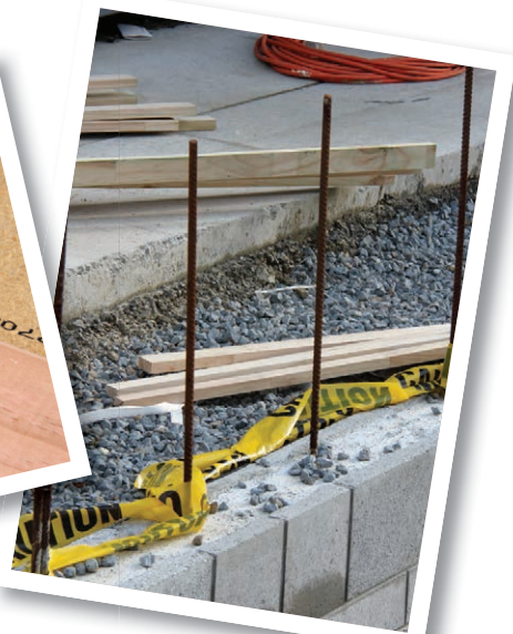
2 RETAINING WALL REINFORCING
