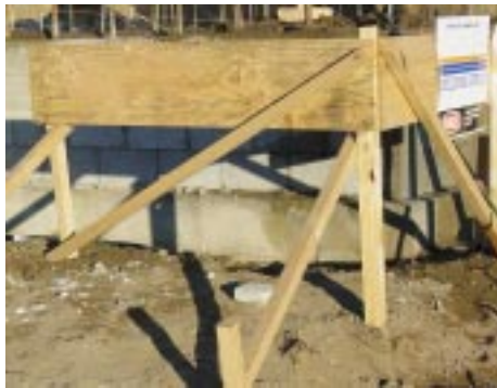
A tall profile at the low end of the site, braced to ensure rigidity
