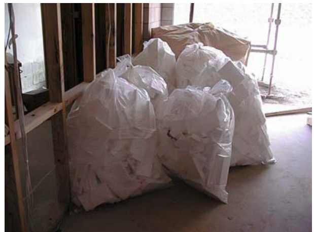
Polystyrene off-cuts can be recycled in some cities – either by the manufacturers or a recycling operator.
