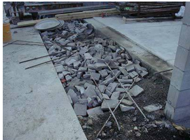
Concrete off-cuts can be incorporated into driveways and hard stand
