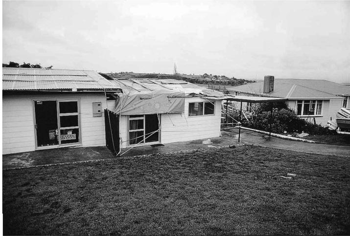
Figure 2 Roof damage caused by high winds in New Zealand (photo courtesy of BRANZ)
