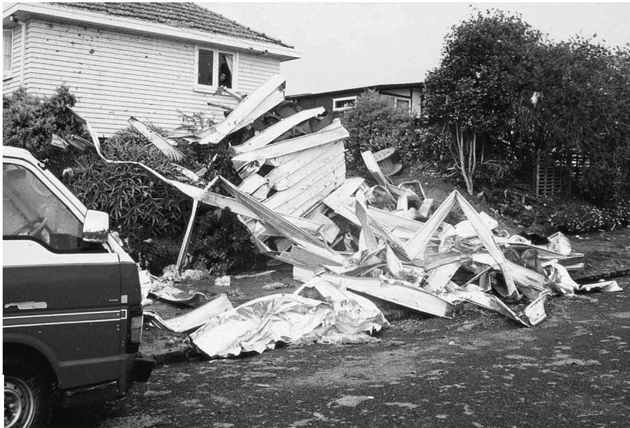
Figure 3 Building damage caused by a landslide triggered by stormwater in an urban area (photo courtesy of BRANZ)
