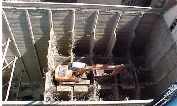
Dismantling the Northern Roller Mills building, Auckland floor by floor (Ward Demolition).
