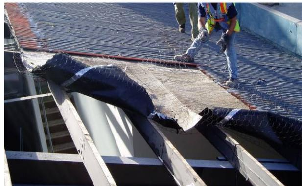
After removing the roofing and bituminous and wire netting underlay from a 1970s commercial building in downtown Auckland, Ward Demolition then cut the 190 x 45 mm rafters into manageable lengths using a chainsaw (for speed), before stacking and transporting them to their used goods saleyard.
