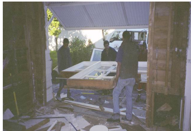
Manual removal of windows (Ward)
