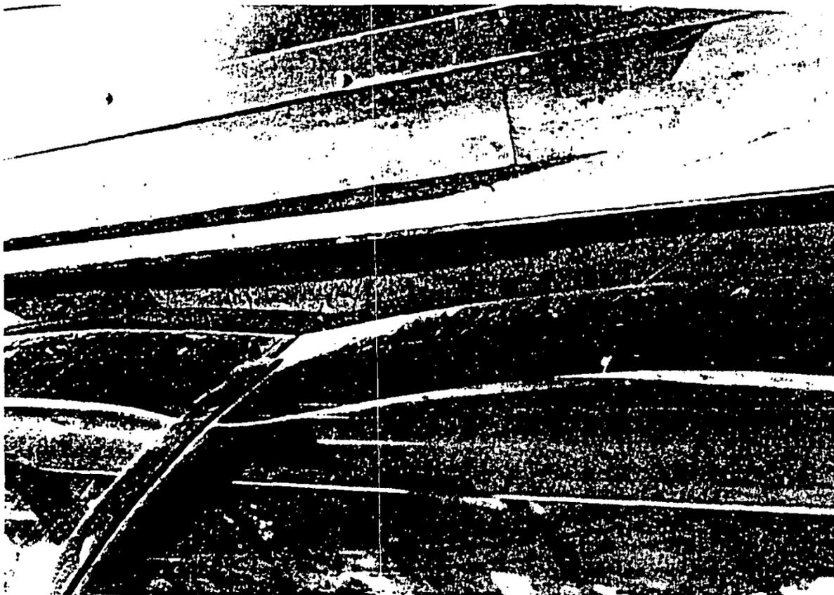
Fig. 4 Polycarbonate verandah detail showing distortion caused by restrained thermal expansion.
