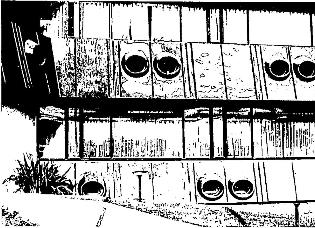
Fig. 3 Weathered GRP panels containing fire-retardant resin.
