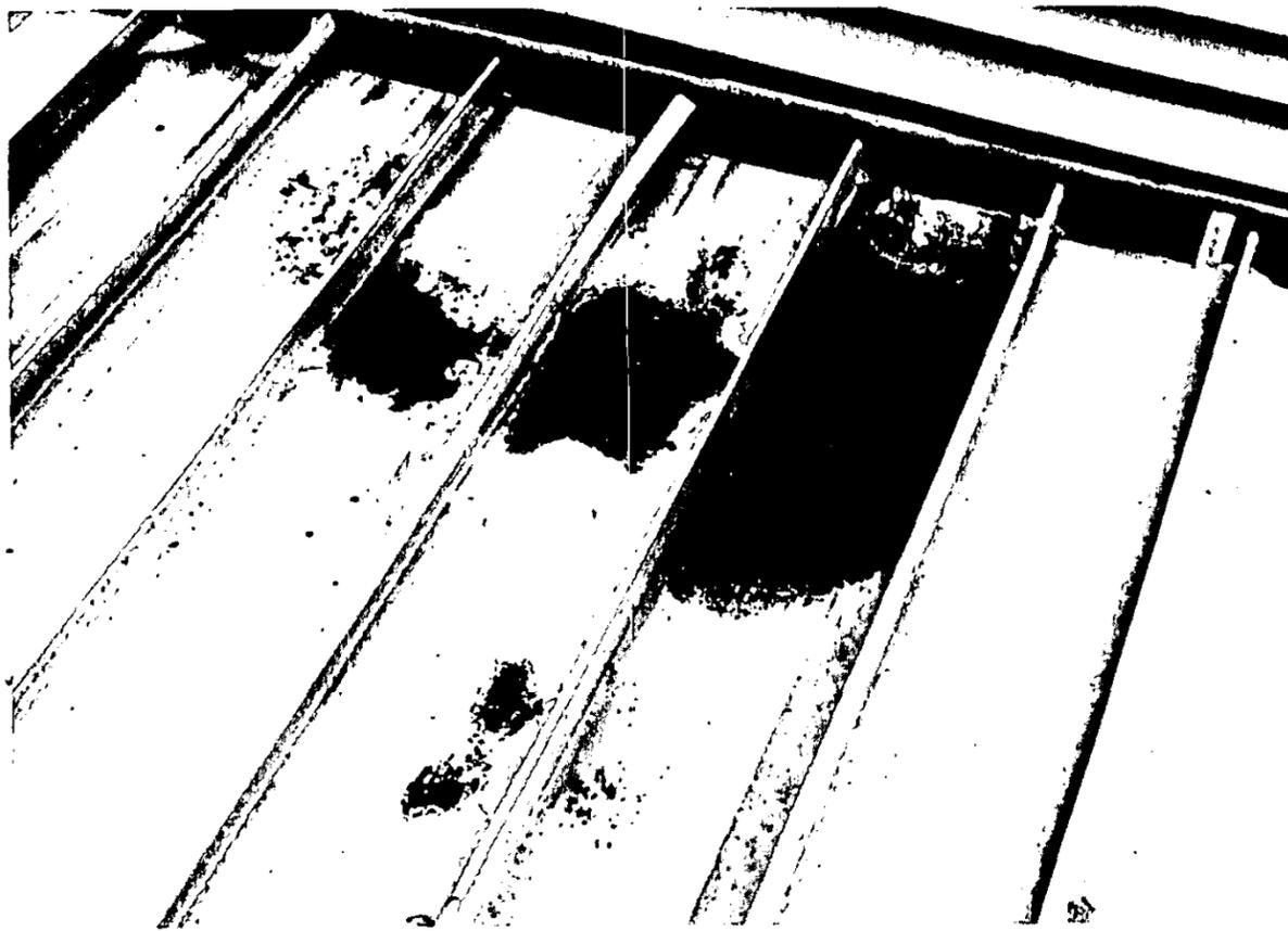
Fig. 1a Degraded PVC plastisol-coated roofing.
