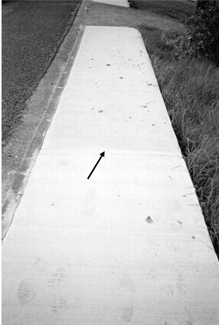
**Figure 4. Transition point between the two concretes.**
