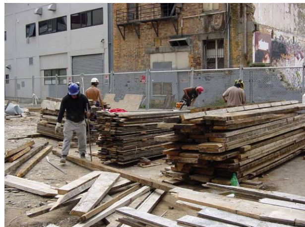
Timber salvage (Ward Demolition).
