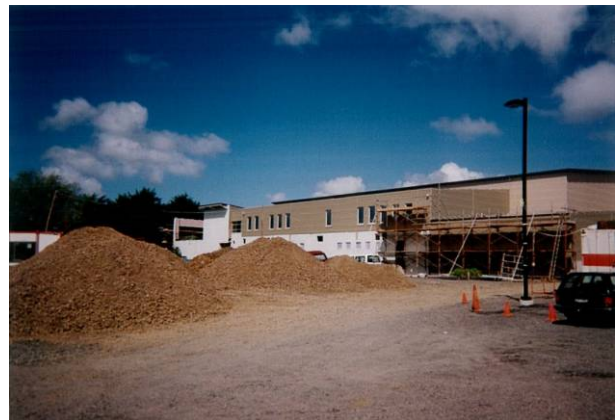
Using crushed concrete aggregate as base course is a simple way to use recycled products.
