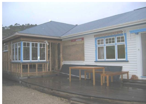
In this home renovation, the original windows were reused in the new extension.
