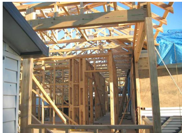
Prefabricated framing means no waste from off-cuts and mistakes.
