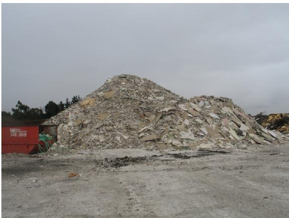
Construction and demolition plasterboard sorted from C&D waste, ready for processing, Crusaders Landscaping, Christchurch.
