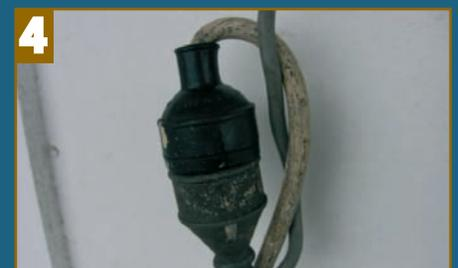
This old way of keeping the leads from parting caused damage. Get the right fitting.
