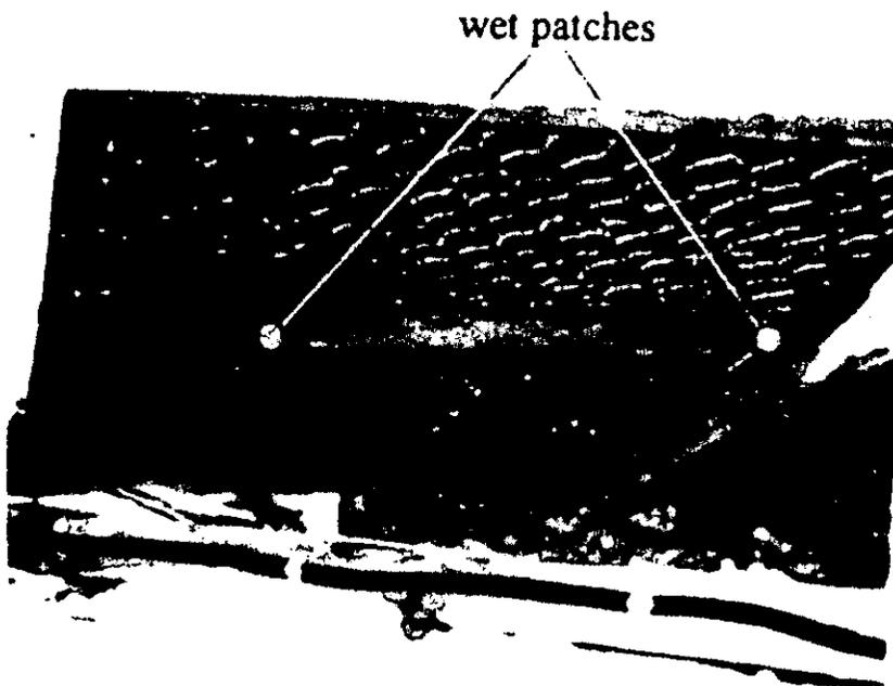
Figure 1 Roof space condensation (survey 1).
