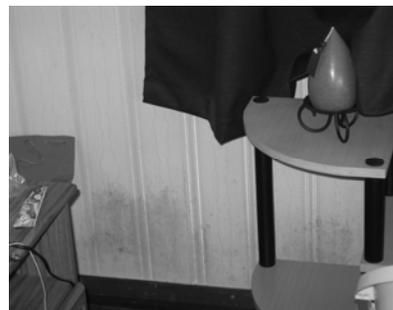
The damp appears to be no worse than a year ago. Attempts to remove the stains have been unsuccessful. The wall linings will be removed in stage 2
