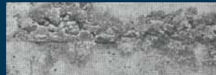
F1. Roughest of all, for use where the finish doesn't matter, such as for foundations where the work will be covered.
