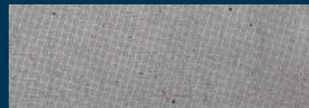
F6: The highest level of finish where appearance and accurate alignment are of greatest importance. This finish is often used in feature panels and also in high-speed water channels to minimise turbulence.
