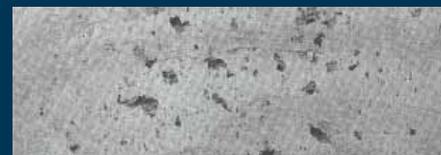
F2. A surface that provides a key for plaster or other thick surface coatings.
