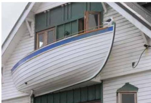
Timber-framed balustrades and parapets are prone to failure, especially if cap flashings are not used.
