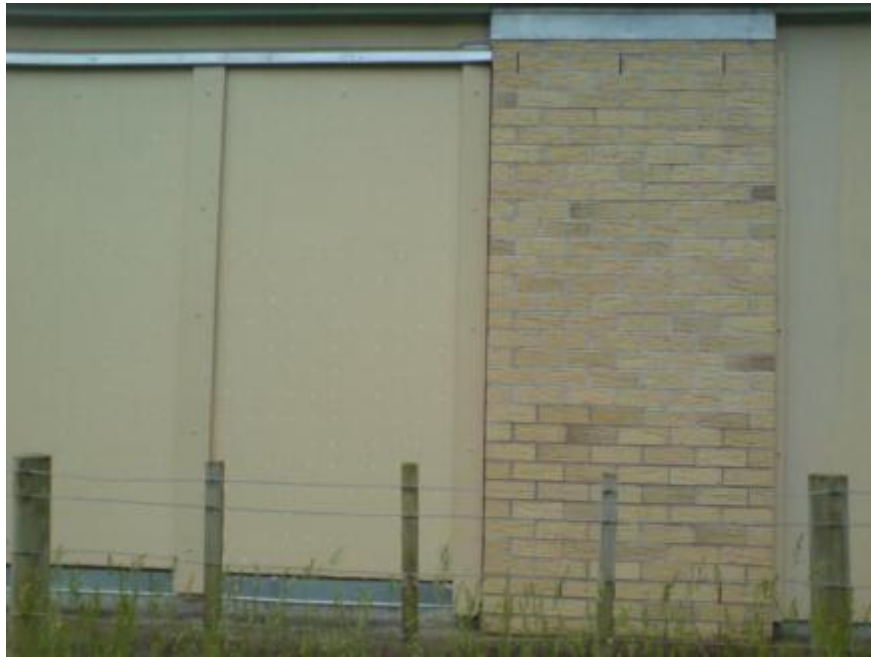
Figure 5: Brick veneer cladding on BRANZ test building
