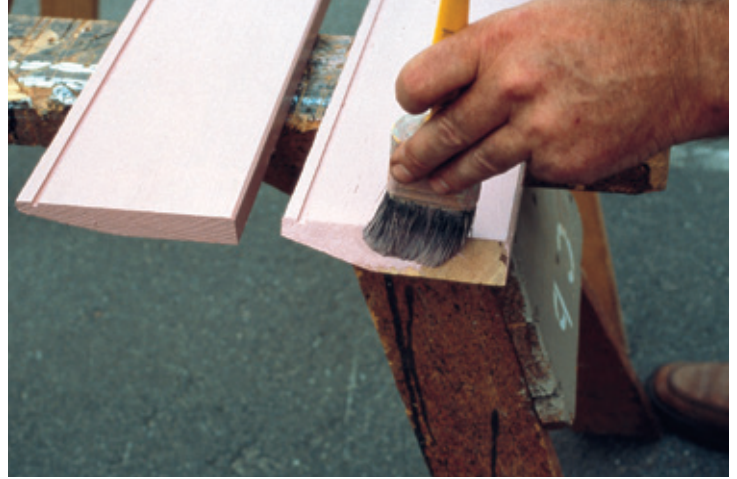
BRANZ recommends two coats of sealer to the cut ends.
