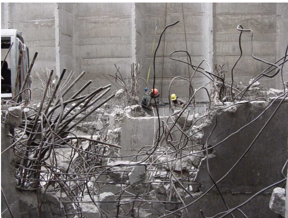
Demolition of Northern Roller Milling Company building, Ward Demolition, Auckland.
