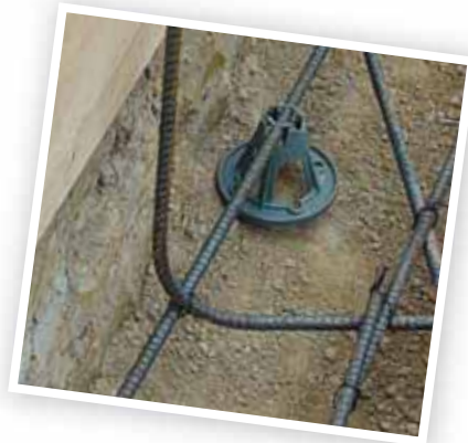
This reo has the right bend diameter but the main bars should never be tied below the stirrups.
