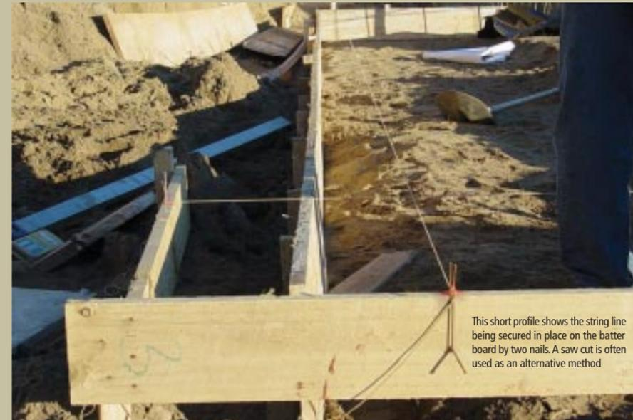
This short profile shows the string line being secured in place on the batter board by two nails. A saw cut is often used as an alternative method
