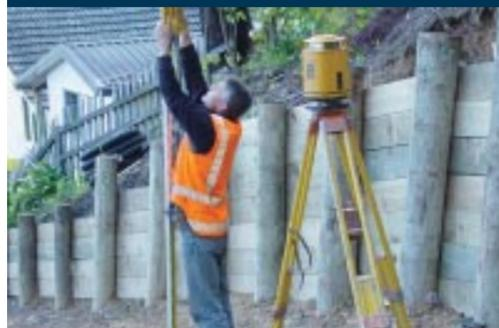
2. The reader unit, attached to a standard measuring staff, is moved up and down until the audible warning sounds are heard. An immovable object, such as a manhole cover, can be used as a set-out datum.
