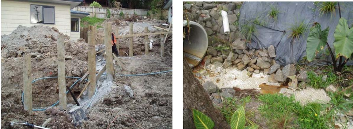
*Figure 2: A typical concrete pollution incident on a construction site – Waitakere City 2006*
