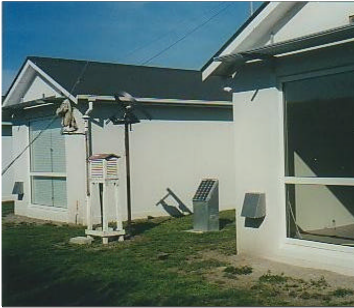
Figure 1. North wall window
