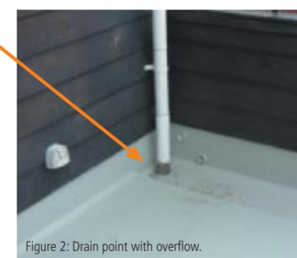
Figure 2: Drain point with overflow.
