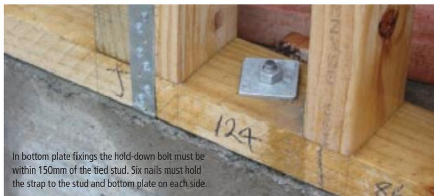
In bottom plate fixings the hold-down bolt must be within 150mm of the tied stud. Six nails must hold the strap to the stud and bottom plate on each side.
