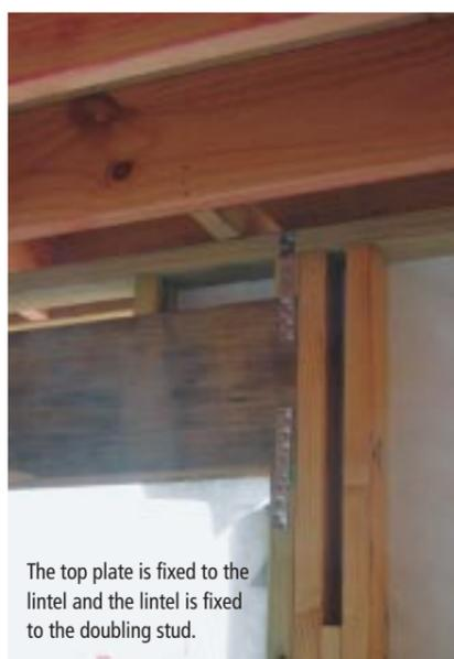
The top plate is fixed to the lintel and the lintel is fixed to the doubling stud.
