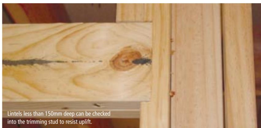
Lintels less than 150mm deep can be checked into the trimming stud to resist uplift.
