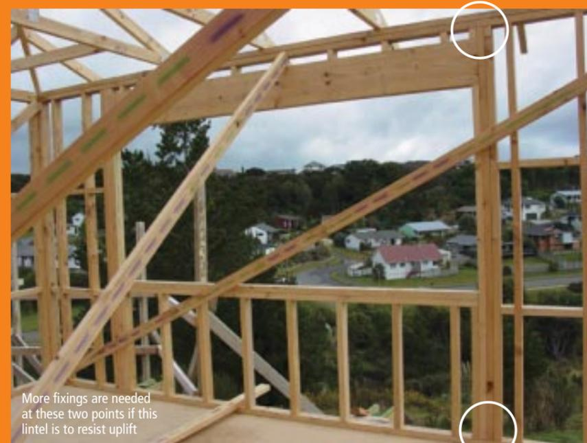
More fixings are needed at these two points if this lintel is to resist uplift
