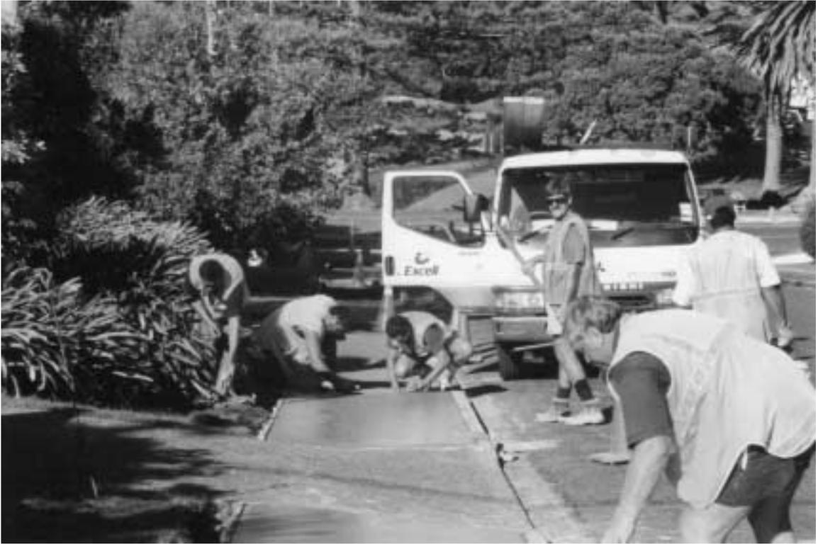
**Figure 9 Finishing Recycled Aggregate Concrete Field Trial**
