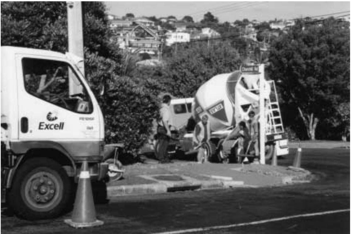
**Figure 8 Placing Recycled Aggregate Concrete For Field Trial**
