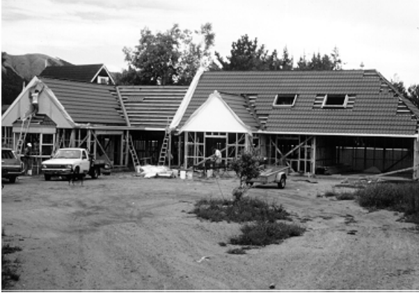
FIGURE 2. Front View of Paraparaumu House during construction
