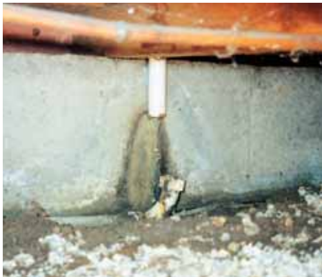
Fix any plumbing leaks before laying polythene.
