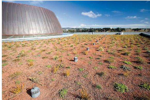
*The civic wing's green roof insulates the building and slows the rate of rainwater flow.*
