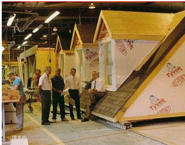
Figure 4: Modular home under construction in a factory (Pinpoint Construction Corp., 2012).
