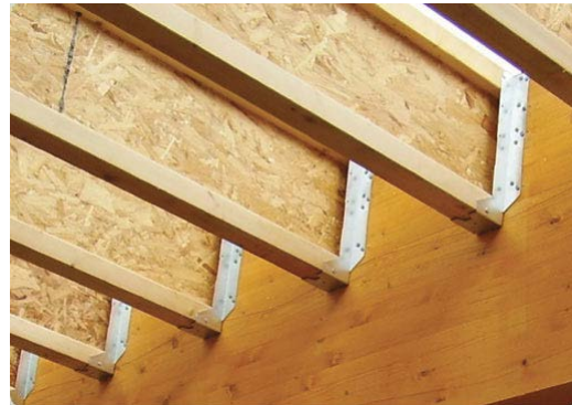
Figure 17: Engineered timber I-joists 'hung' off a laminated veneer lumber (LVL) beam (James Jones and Sons Ltd, Timber Systems Division, 2012).
