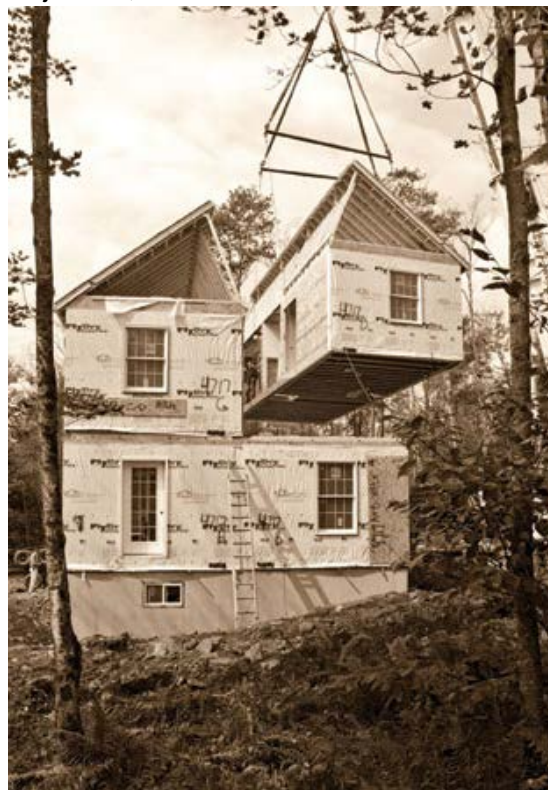
Figure 39: The hinged roof enables modular manufacturers to include steeper pitches without exceeding transportation height limits. Image: Ellen McDermott (Gorman, 2012).
