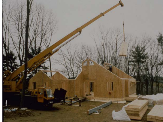
Figure 32: SIPs house under construction (Sunlight Homes, 2013).
