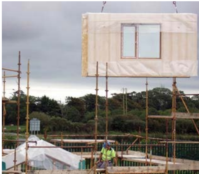
Figure 21: Closed panel wall being craned into place (The Timber Frame Company, 2013).
