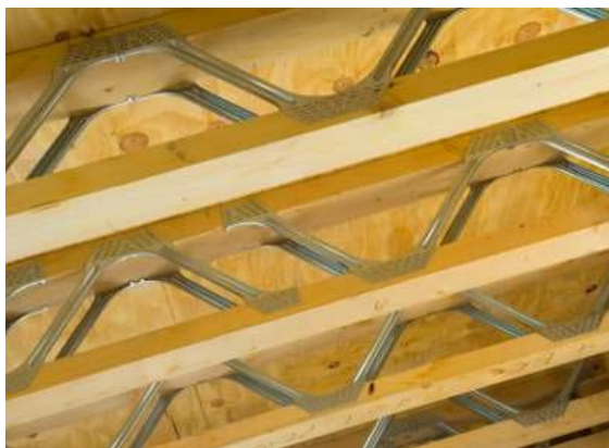
Figure 18: Engineered timber I-joists often employ steel as a webbing material (Timber Engineering Europe Ltd, 2012).
