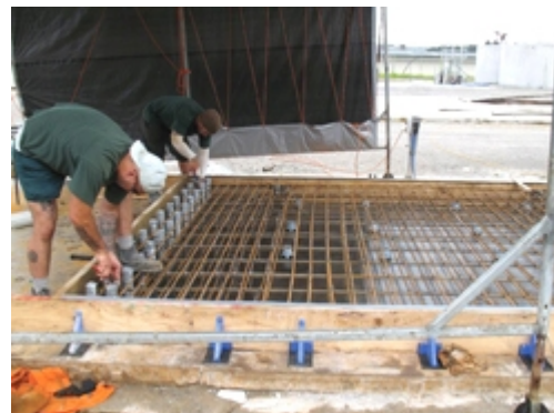
Figure 24: Workers casting concrete panels in a make-shift factory (Department of Corrections, 2009).
