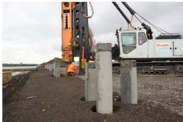
Figure 14: Helical pier piles are screwed through the ground into a stable substrate (Basement Systems, 2012). Figure 15: Precast concrete piles are driven into the ground (Simplex Westpile, 2012).
