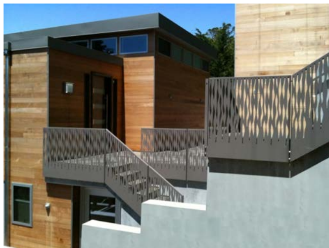
Figure 6: Laser-cut steel panel balustrades (BokModern, 2012).
